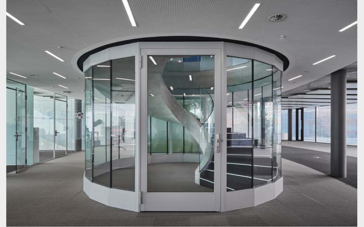
Maison de la Paix, Geneva, Switzerland Single and double-leaf fire resistant doors – forster fuego light EI230 Glass elements connected with butt joints – forster fuego light EI230/EI260 Image: Damian Poffet
